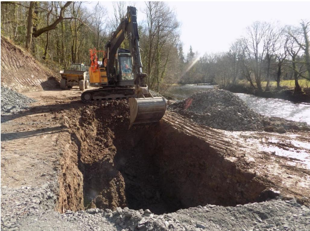
Temporary piling mat constructed in advance of piling rig arriving at site.
